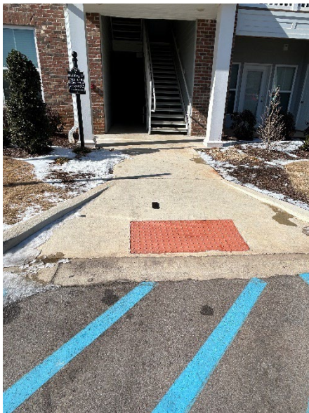
Figure 14: Slope on curb cut entering Building 17
