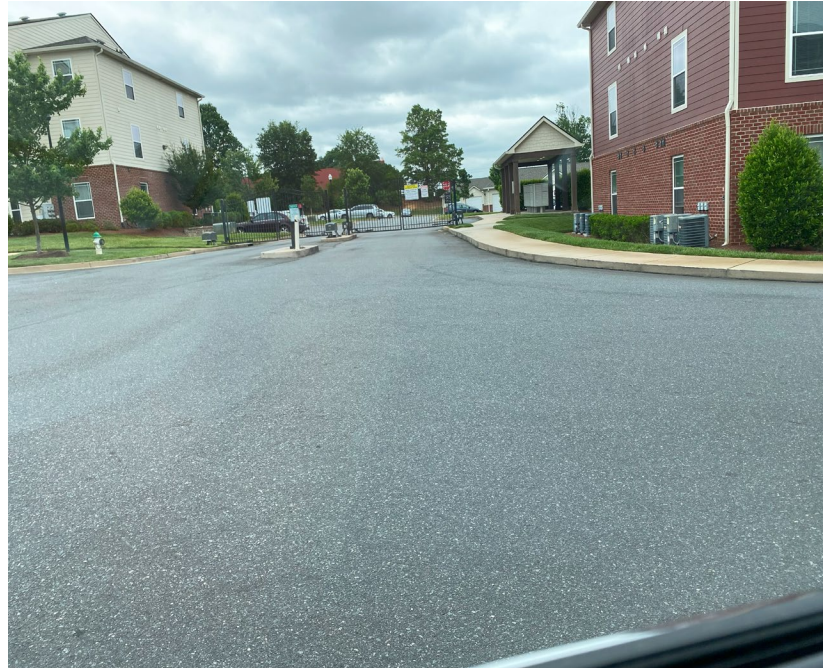
Figure 17: The route leading to the mailbox kiosk containing mailboxes at the Revere at Lake Wylie does not contain a curb cut.
