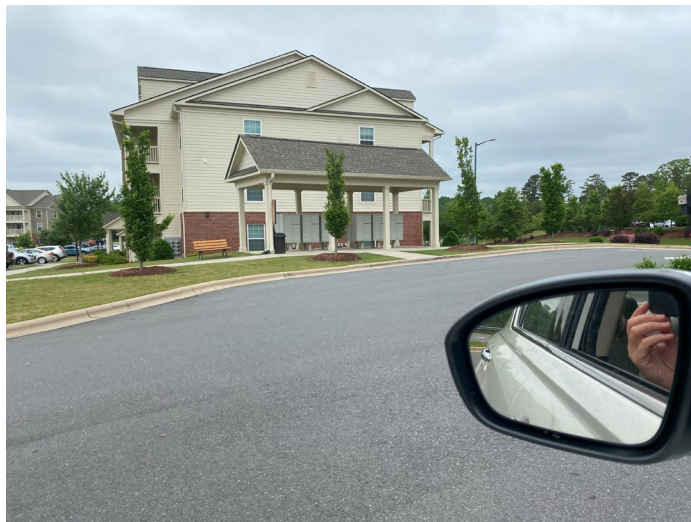
Figure 19: The route to the mail kiosk by the second gate at Revere at Tega Cay does not have a curb cut.
