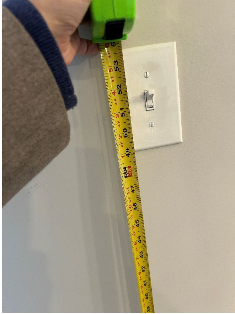
Figure 32: Operable part of light switch at Revere at River Landing above 48 inches
